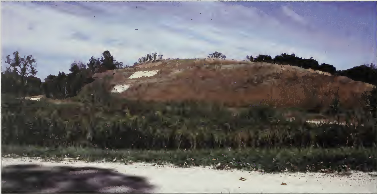
Figure 10 View of the Mineral Point roaster waste after reclamation circa 2004.
